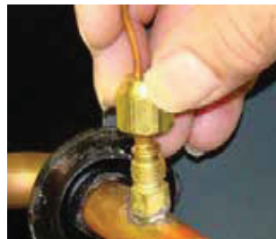
B. Screw flare nut on TXV equalization tube on to the Schrader valve stem.
