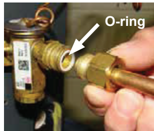
III-9. Remove the additional Teflon O-ring seal from the box and place on the shoulder just inside the TXV inlet port. Screw the nut attached to the stub-out portion of the flowrator body onto the inlet port of the TXV.
