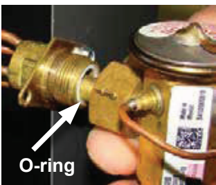
III-6. After ensuring that the Teflon O-ring seal is still in place inside the flowrator body, screw the female swivel nut onto the flowrator body.
